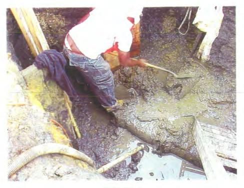
SITE NO. 7 EXCAVATING 8" CAST IRON WATERLINE
